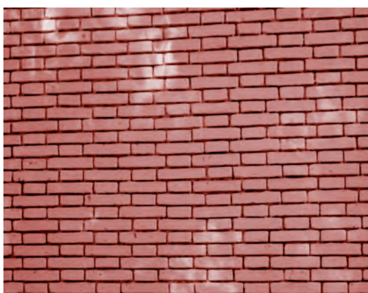
(a) Brick wall
